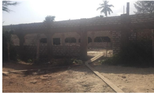
our dining and kitchen building in progress
