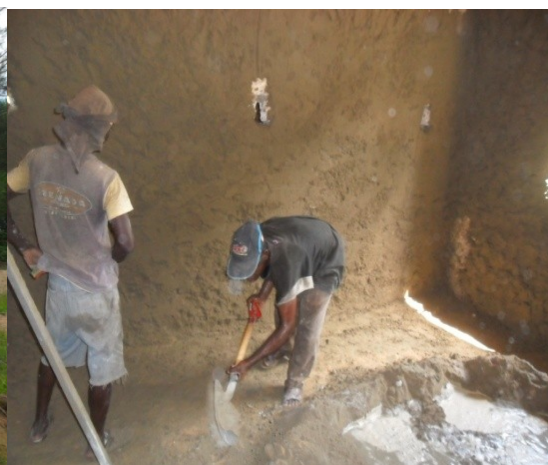
Inside plastering in progress
